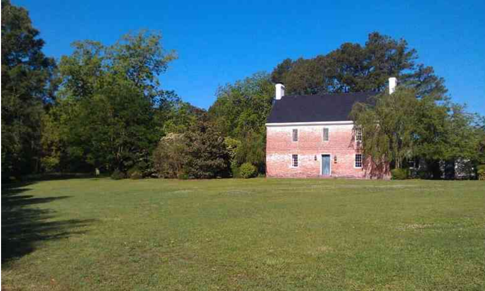
Figure 9: Example of Unique Historic Property in Camden County
