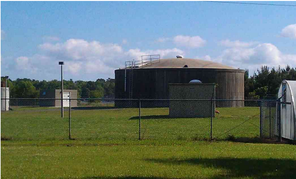
Figure 7: Proposed Large Scale Developments Offer an Opportunity to Expand Utility Infrastructure in Camden County
