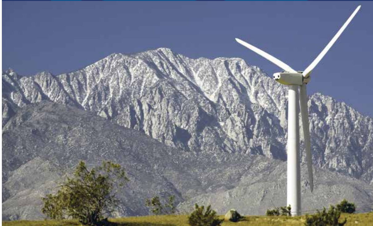
DILLON WIND POWER PROJECT, PHOTO BY IBERDROLA RENEWABLES, INC., NREL 16105
