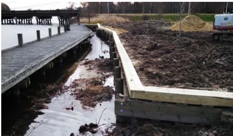
A new bulkhead will protect the park's shoreline from erosion.
