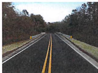
Muddy Creek Road Bridge
