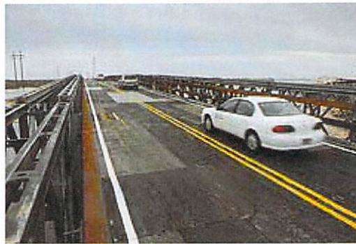
Current temporary bridge on N.C. 12 at Pea Island.
