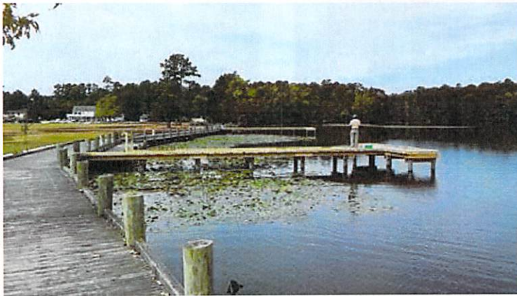
Two 50' piers provide access to deeper water for fishing. Photo: Mark Powell
