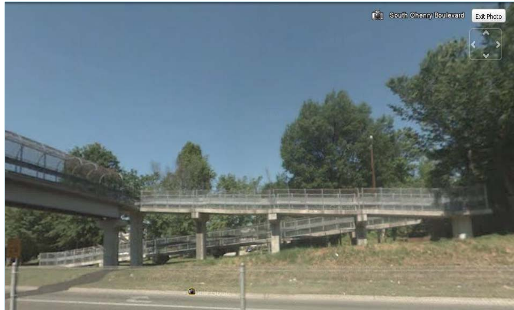
Figure 1 - ADA Compliant Approach Ramps on Pedestrian Bridge in Durham, NC
