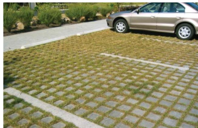
Incorporating stormwater management techniques into parking lots can include requiring landscaping and disallowing curbs and gutters so that water can flow into, not away from landscaped areas (left) and incentivizing the use of alternative pervious paving that allows water to permeate where it falls (right).
