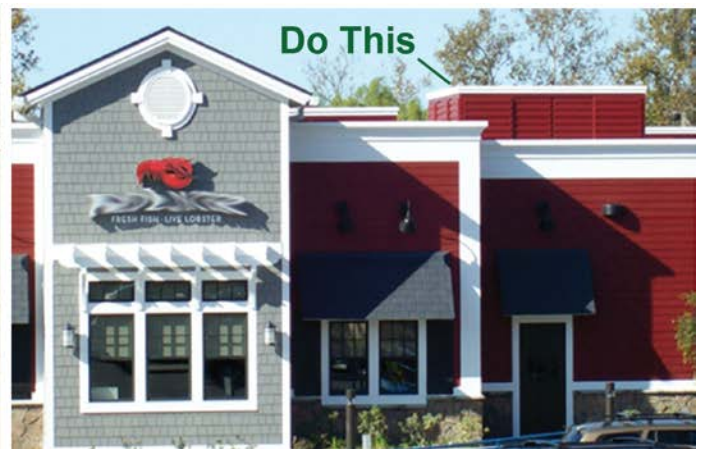
FIGURE <>: ROOFTOP EQUIPMENT SCREENING
