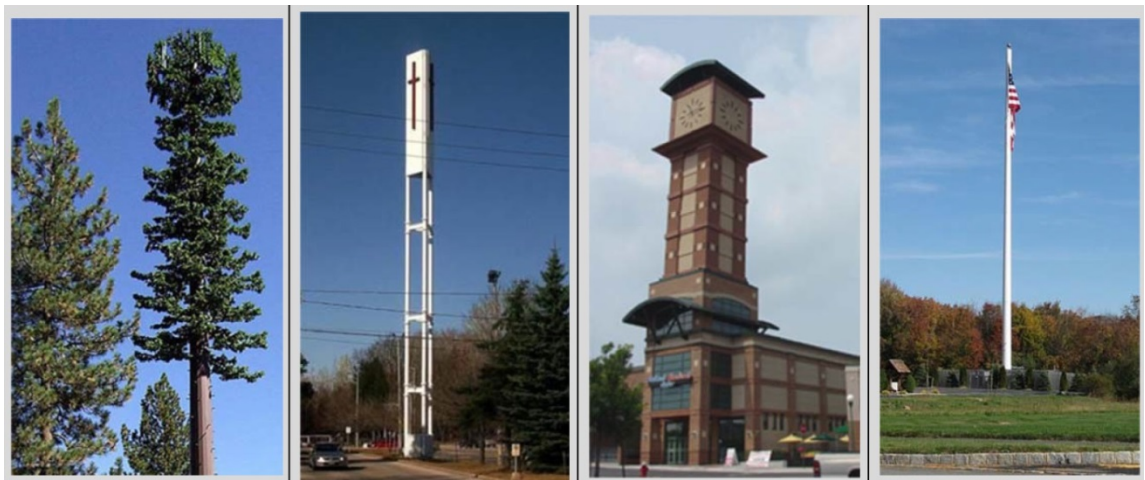
FIGURE <>: CONCEALED TELECOMMUNICATIONS TOWERS
