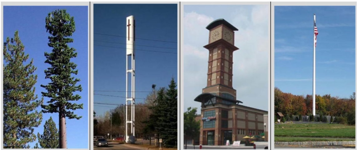
FIGURE <>: CONCEALED TELECOMMUNICATIONS TOWERS
