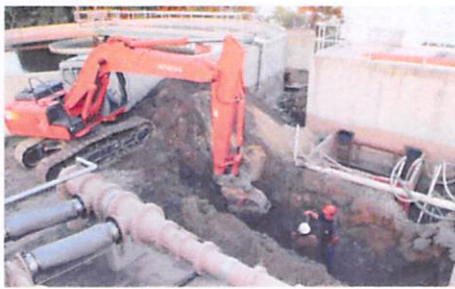
Elizabeth City's Rogerson WWTP
